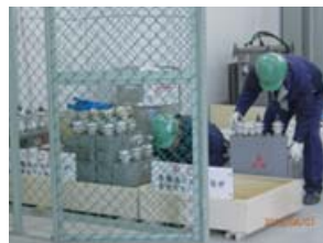
Removal of equipment containing PCBs (Fujieda plant of CPMC)
